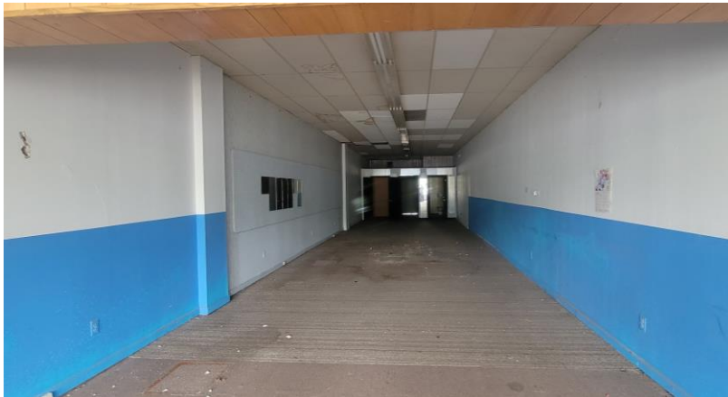
Photo 5: Interior of Former Dry Cleaners
