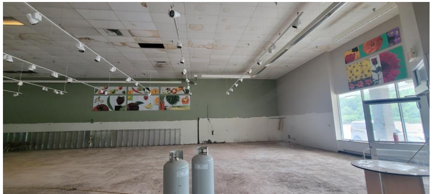
Photo 2 – Anchor Space under Renovation
