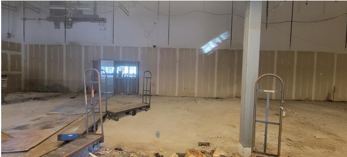
Photo 11: Interior of Anchor Store under renovation
