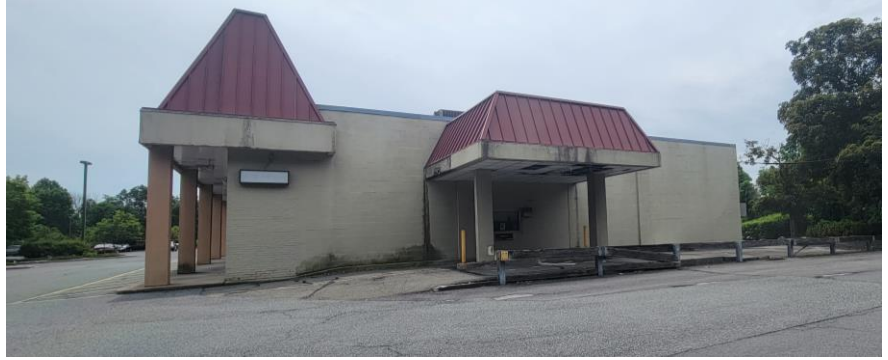
Photo 1: Exterior of Bank and Drive-Thru
