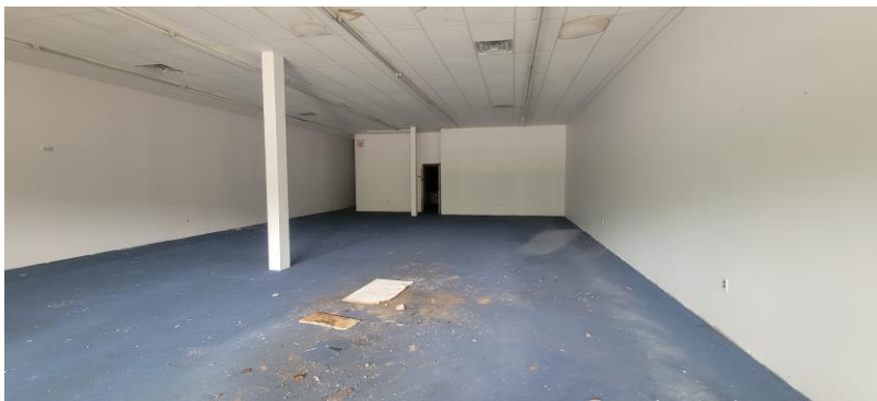
Photo 6: Interior of Former Video Rental
