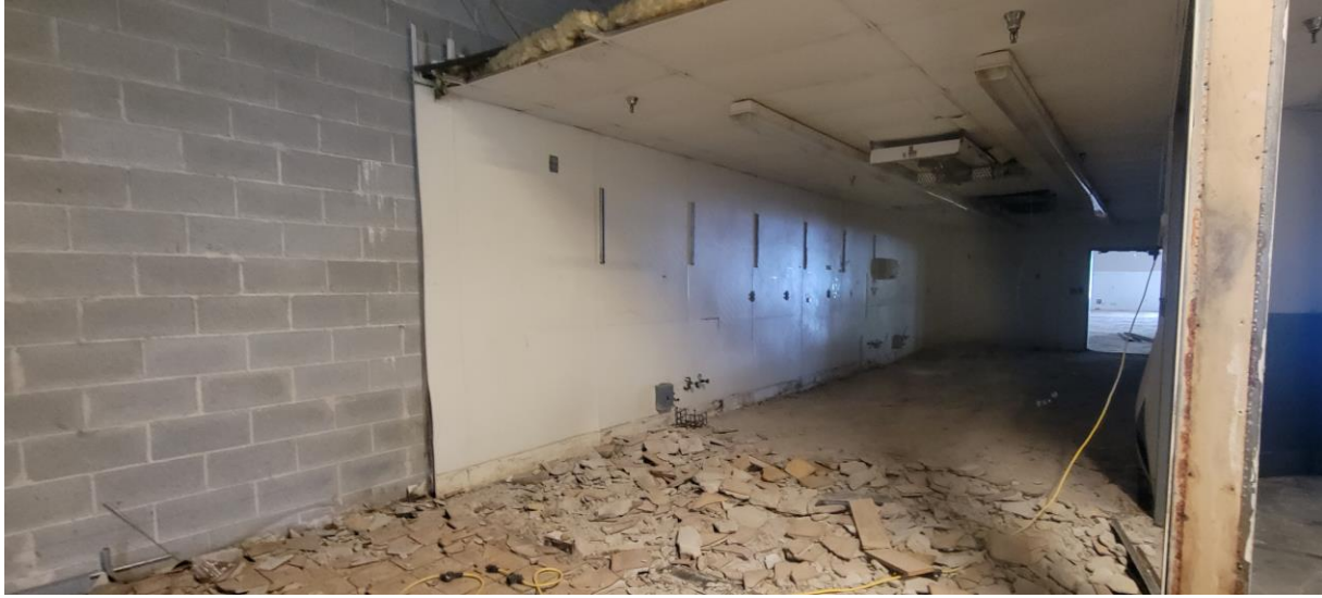
Photo 10: Interior of Anchor Store under renovation
