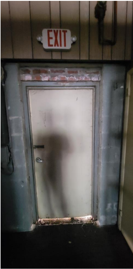
Photo 12: Rear entrance to Former Dry Cleaners
