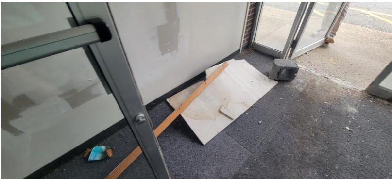
Photo 17: Former Bank Foyer
