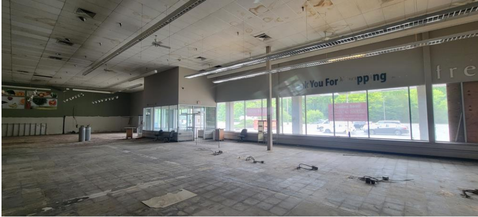
Photo 7: Interior of Anchor Store under renovation
